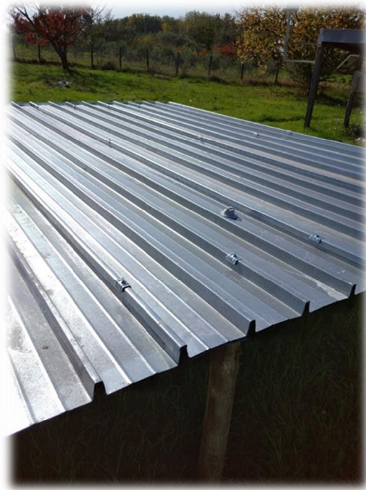
Figure 7. The steel roof (benchmark).
