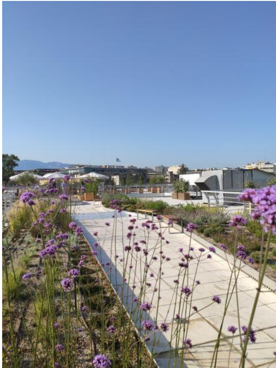
Figure 12: The extensive biodiversity green roof
