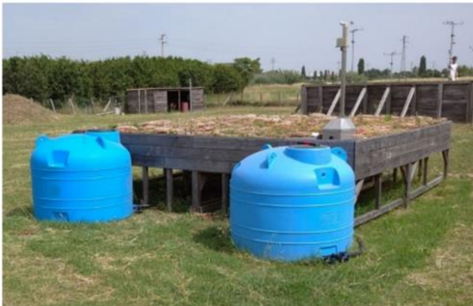
Figure 4. The BGR case study in Viterbo (Central Italy)
